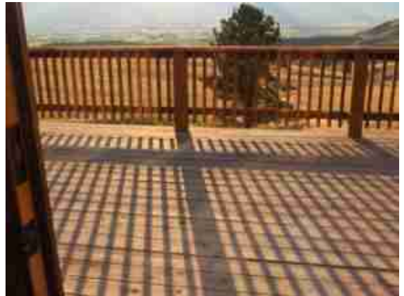
(1756 Sapphire Ranch Trail west side deck.) i262854AM
