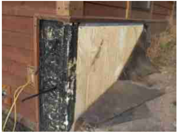
(1756 Sapphire Ranch Trail tar paper pealed loose.)
