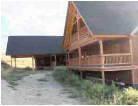
(1756 Sapphire Ranch Trail view of front from north side.) i262854R
