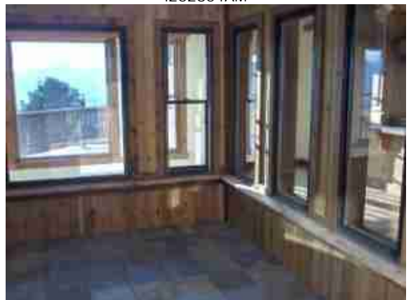
(1756 Sapphire Ranch Trail solar room.) i262854AO
