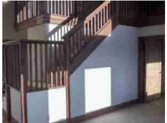
(1756 Sapphire Ranch Trail stairs to master bedroom loft.) i262854AC
