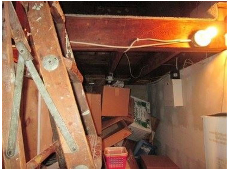
storage area hazard
