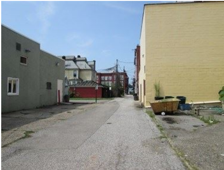
adjacent property: alleyway next to right side of property, taken from across diamond street, north side
